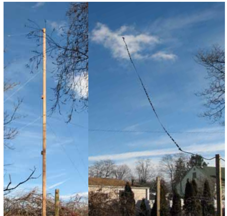
(Left) The mast raised and guyed. (Right) The antenna and feedline.
